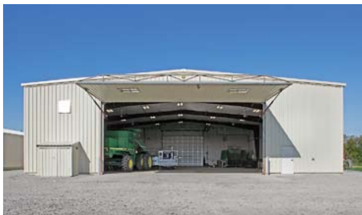
The 8,000-square-foot metal building was completed in a speedy three months and features a one-piece, 40' x 18' hydraulic door on one end of the building.
